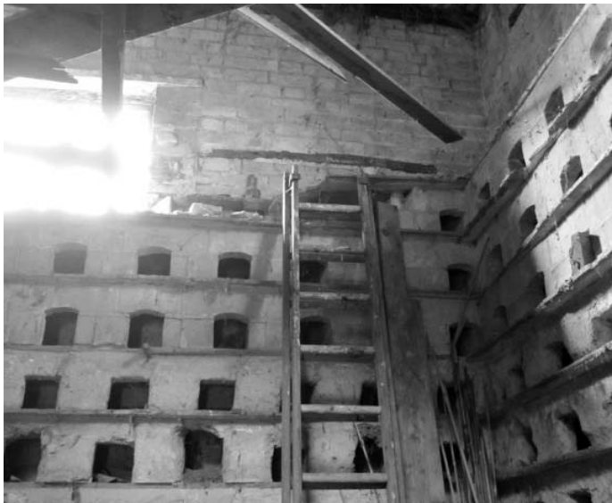
Interior of Hemingford Grey dovecote with nesting boxes.
