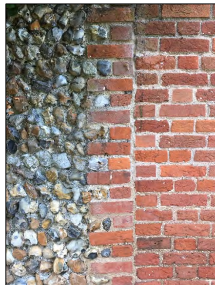
Fig. 2. Looking NW at exterior of SE wall: the four-sided garden has brick walls in Flemish bond while the three sided garden wall is flint in this aspect. The brick join was not well keyed in.
