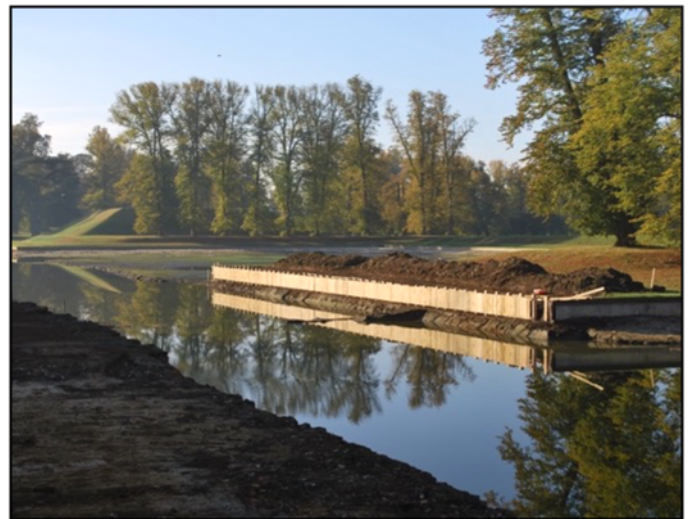
Figure 18. Oak boarding used to revet the canal banks.
