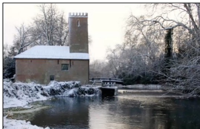
Figure 25. Euston water mill built 1731 by Kent; the tower houses a large water tank supplying the Hall.
