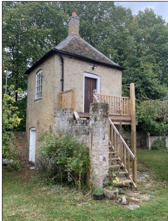
Figure 4. Barnes House gazebo. North elevation has stairs to first floor room while east elevation has door to ground-floor room and first-floor window facing downstream.
